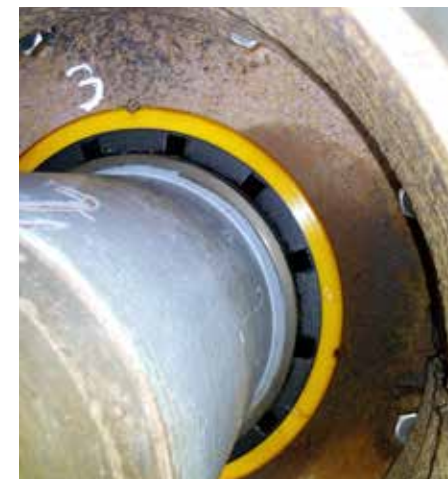
Installation of Thordon Bearings' RiverTough bearing to Impala Zambrano
