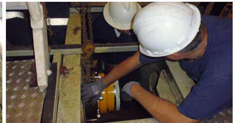
The Delta Marine and River and Thordon Service technicians installing a Thordon TG100 seal on the Impala Zambrano
