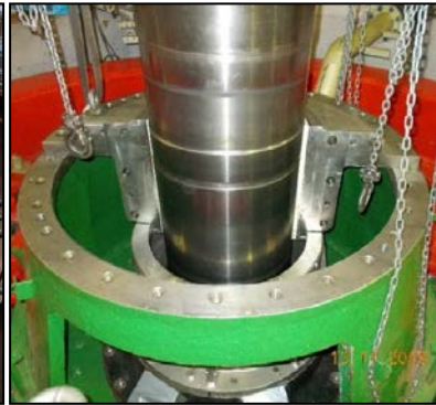
Figure 8 - Bearing Installation
