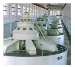
As a result, the committee recommended that Fengman Hydropower Station continue to use Thordon SXL which ran without issue for the next 11 years before the turbines were completely replaced. It was the first time a Chinese hydroelectric plant has installed a Thordon SXL main guide bearing.
