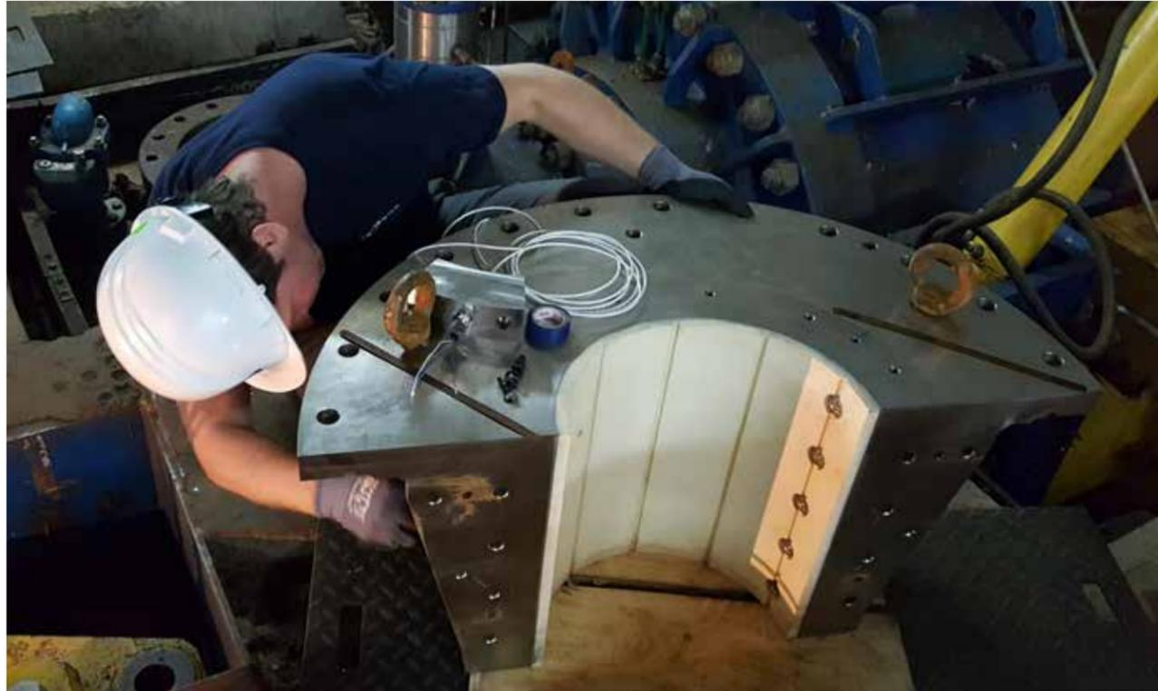
A member of the Global Service & Support team installing an SXL guide bearing in a split stainless-steel housing
