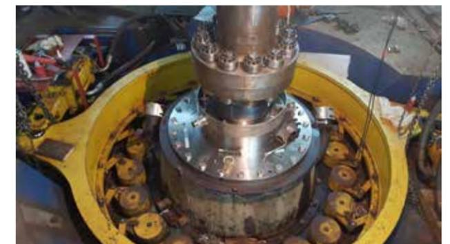
The Stage-1 turbine began operations in March 2018 with the new water lubricated bearing and shaft seal assembly. Since no additional oil lubricating system is needed, Andritz Hydro and WBSEDCL will benefit from a reduction in operational costs, while the maintenance requirement will be optimised with a Thordon shaft seal positioned above the bearing for easier access. ☺
