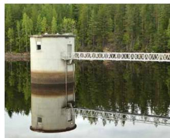
The 1967-comissioned Noppikoski Hydropower Plant operates on the Oreälven river in central Sweden with an installed capacity of 10MW and annual power output of 33GWh.
