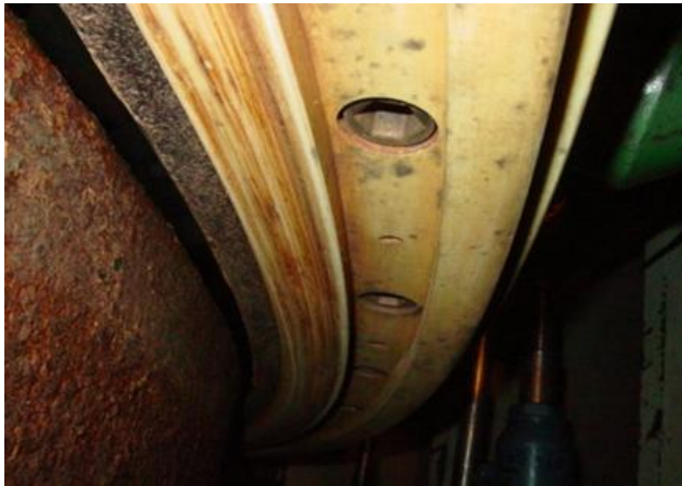
Figure – 9: Sealing faces after cleaning
