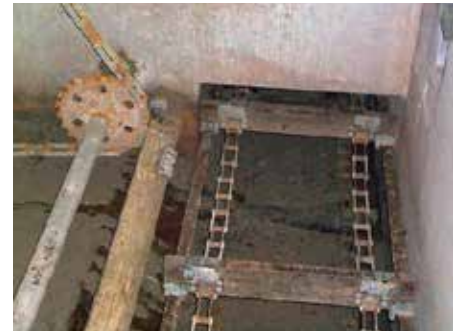
Grit Chamber Scraper Apparatus
