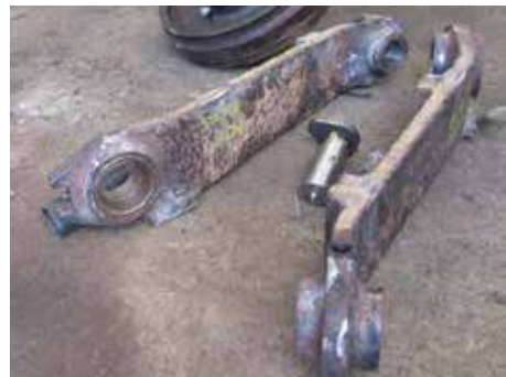
Elevator Support and Existing Steel Bearings
