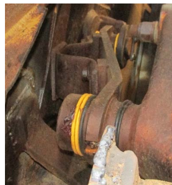
ThorPlas installed with O rings
