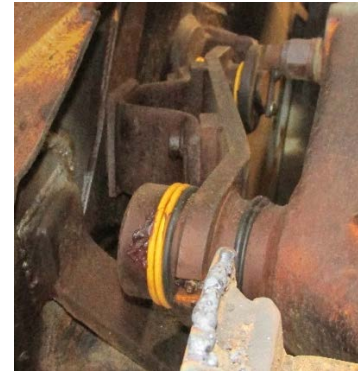
ThorPlas installed with O rings
