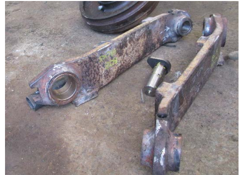
Elevator Support and existing Steel Bearings
