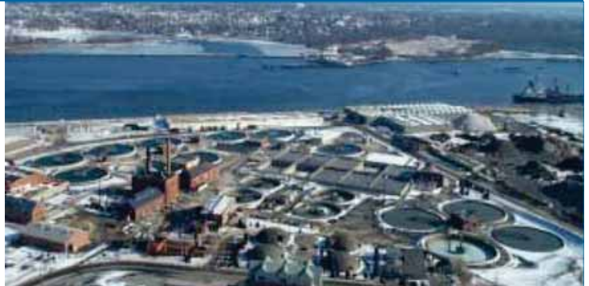
Fields Point Wastewater Treatment Facility
