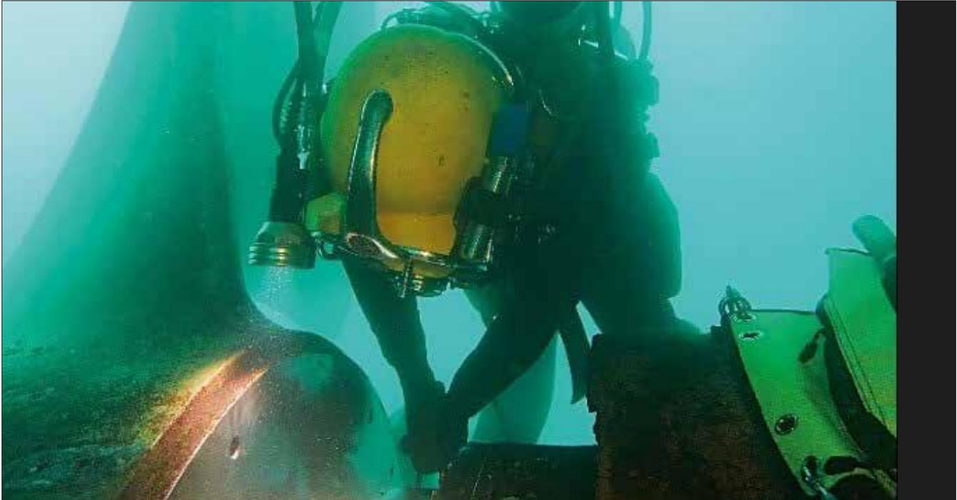
Recently, Hydrex diver/technician teams were deployed to ships in Belgium and Spain for stern tube seal replacements. The first operation took place in Algeciras on a 225-meter container ship, while the second was carried out in Antwerp on a 295-meter RoRo vessel.
