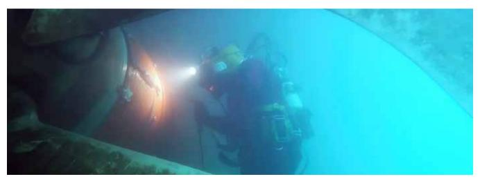
Earlier this year our diver/technician teams carried out a double underwater stern tube seal repair on a RORO ship berthed in Port of Burnie, Tasmania. The ship was leaking oil, making an on-site repair necessary. Using two Hydrex flexible mobdocks simultaneously the team was able to carry out the entire operation on-site and underwater, saving the owner an expensive and time-consuming trip to drydock.
