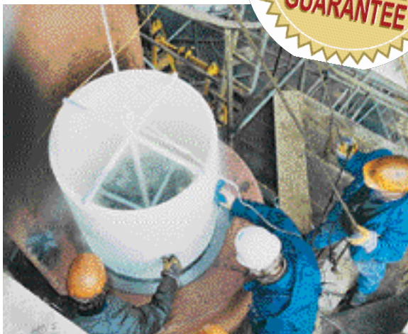
SXL Rudder Bearing Installation
