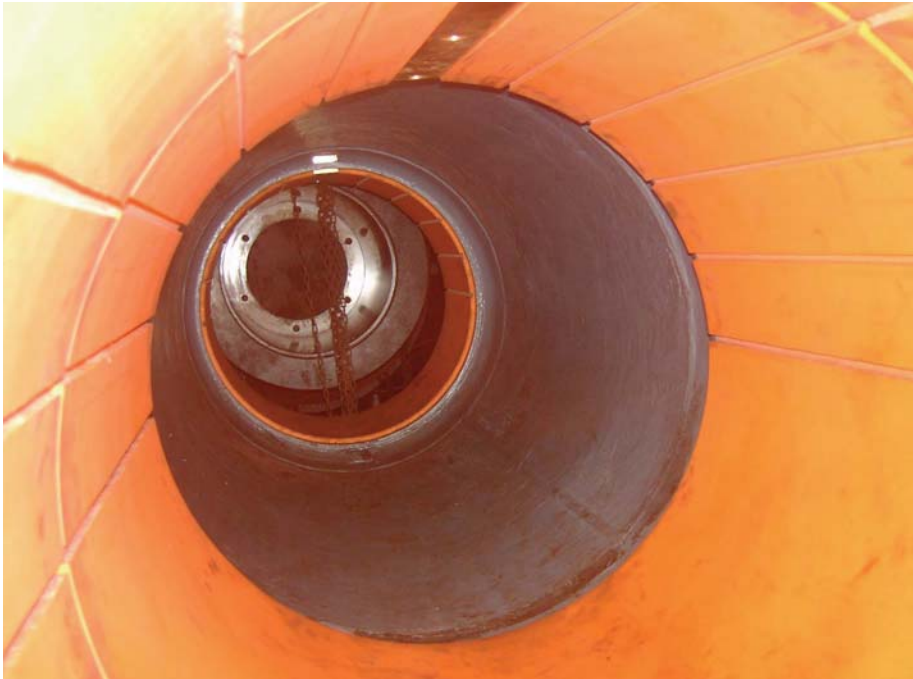
COMPAC fitted to stern tube
