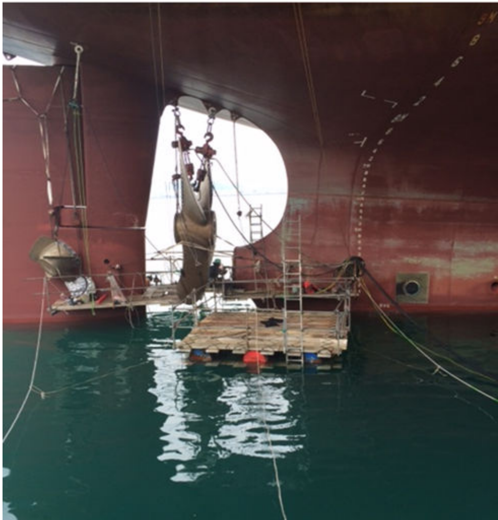
FIGURE 1 Forward Ballasting of a vessel for shafting repairs
