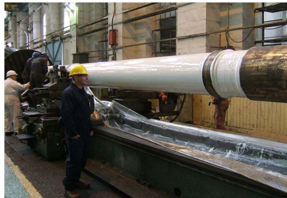
Figure 8: Epoxy shaft coating
