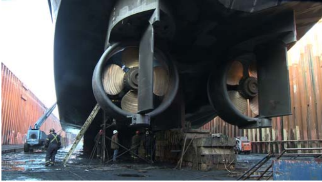
Figure 7. Propeller shafts installed
