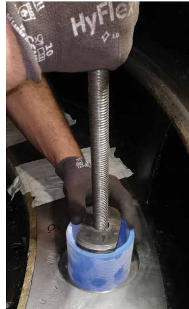
ThorPlas-Blue wicket gate bearing being press-fit into place
