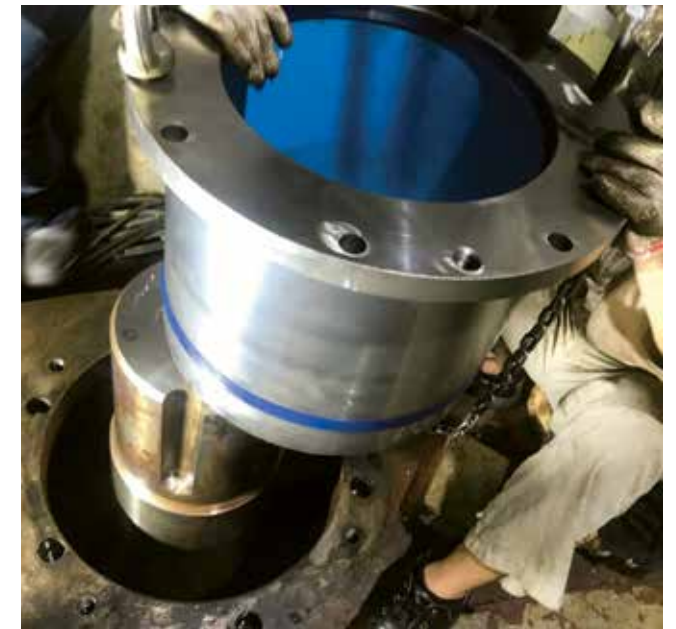
Bearing installation at the Son La Hydropower plant
