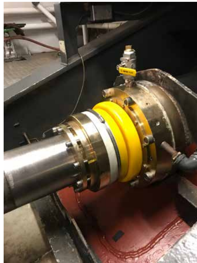
A new TG100 seal was specified and installed
