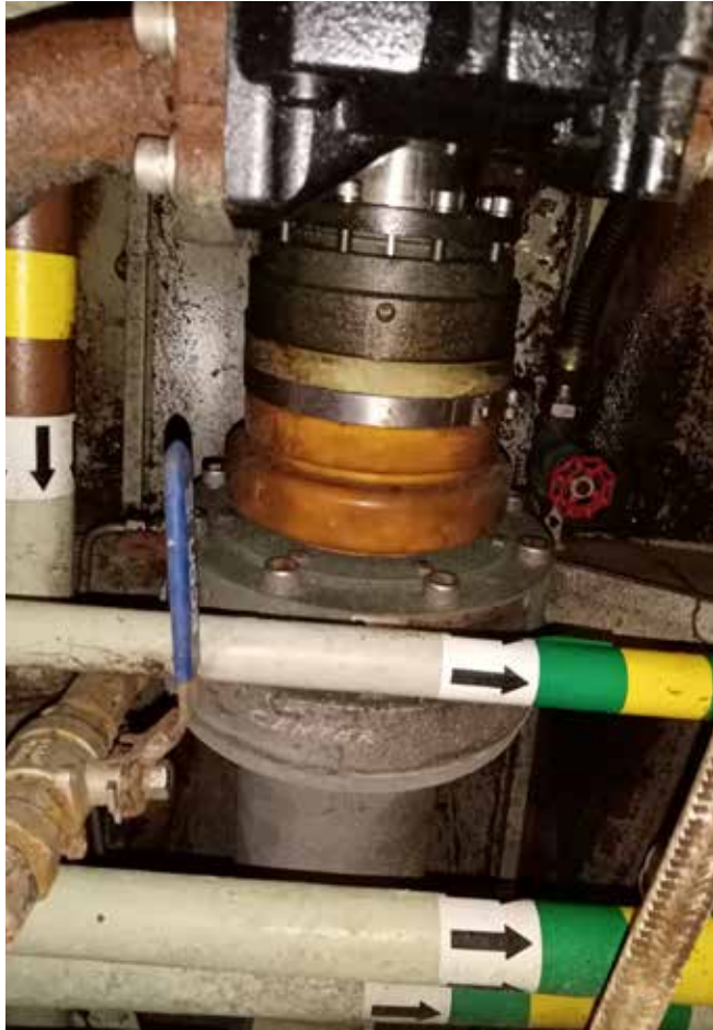
TG100 seal after 3.5 years of stellar service on the Global Tiger
