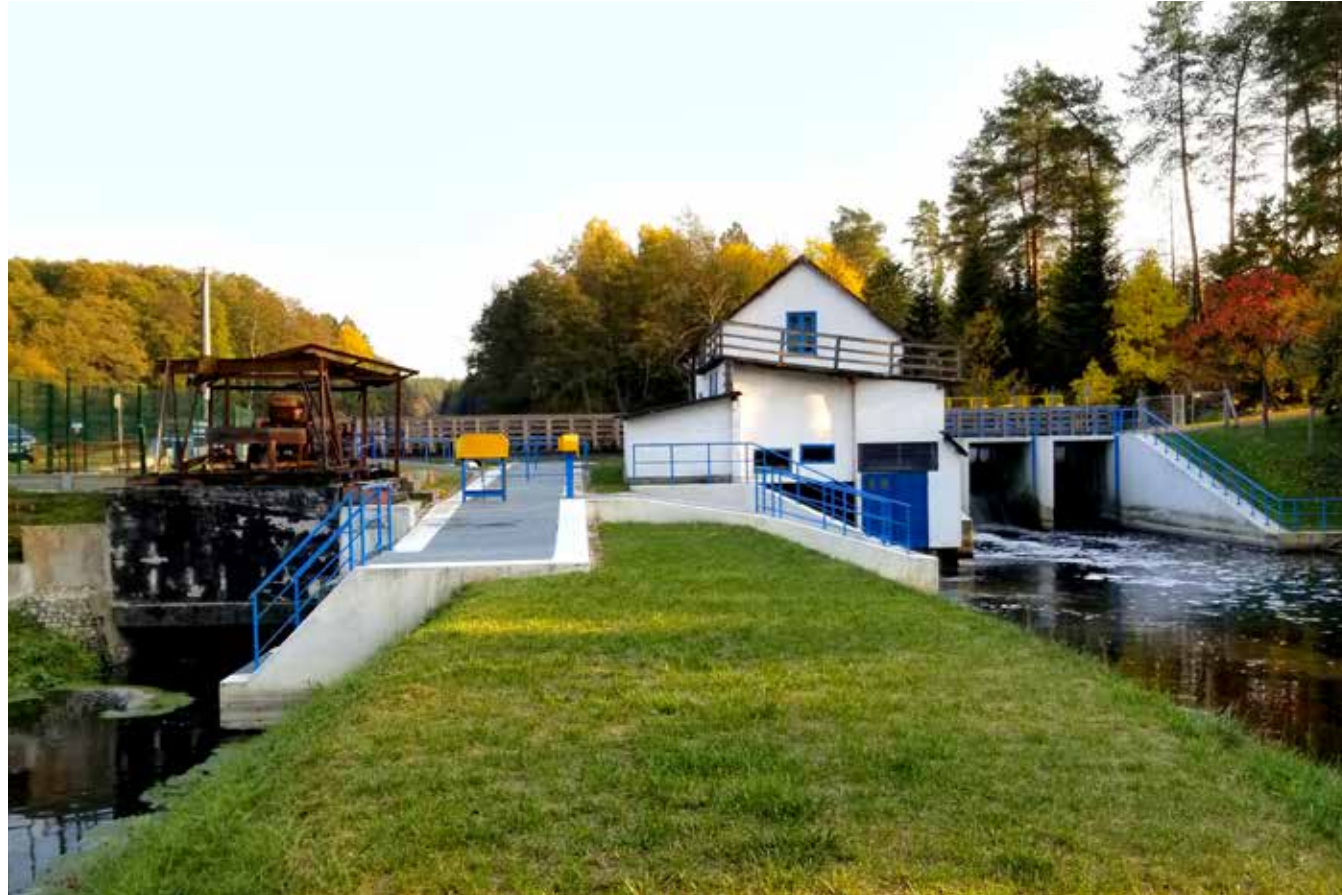
Struzyska Hydro Plant in Pila, Poland
