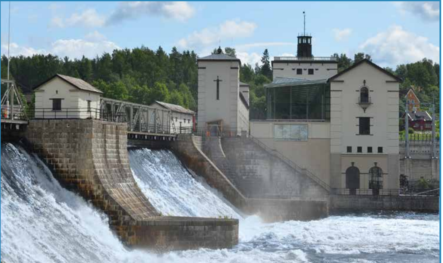
Raanaasfoss 1 Hydro Plant in Norway
