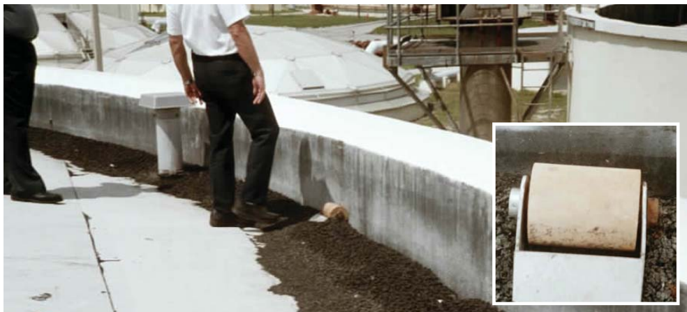
Thordon SXL Tank Roller Application at a Florida Sewage & Wastewater Treatment Facility
