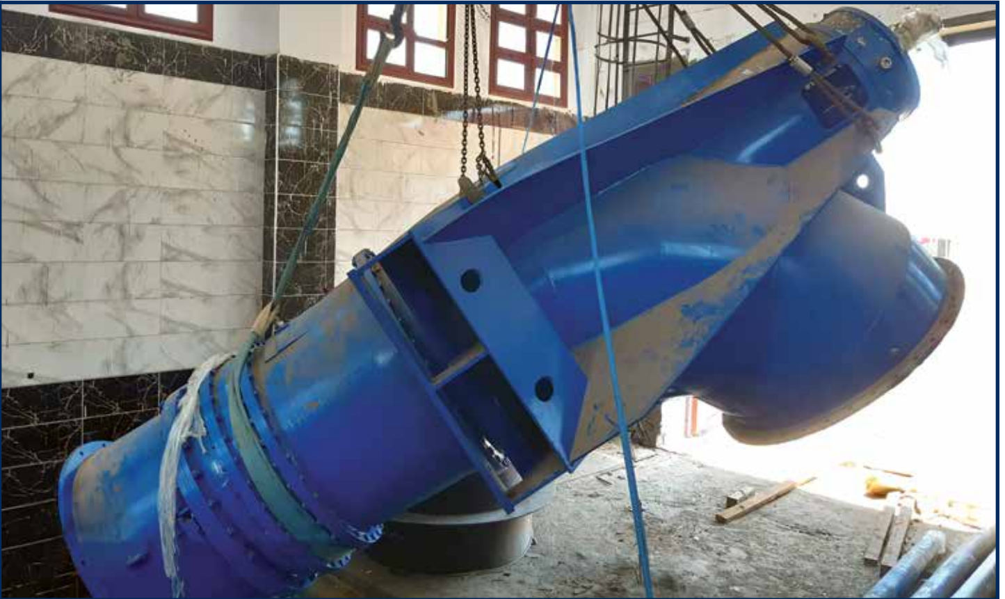
SIGMA incline pump fully assembled with Thordon's pump bearings and ready to be installed.
