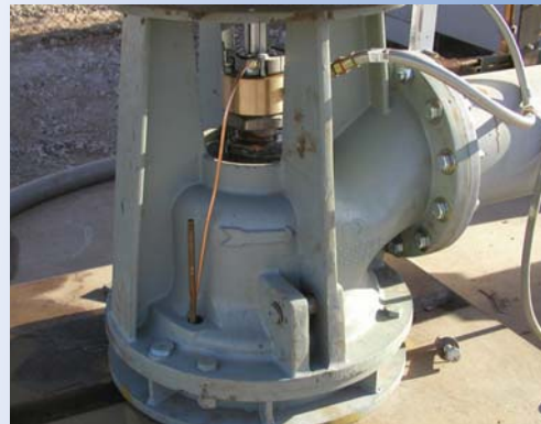
Water Lubricated SXL Bearings Installed In SRP Deep Well Pump, Arizona, U.S.A.
